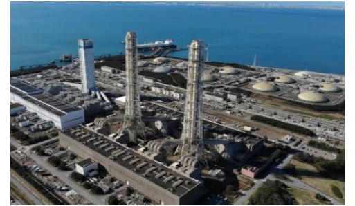
Our Thermal Power Plant (Aerial View)
