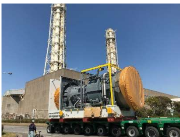
Transporting new gas turbine rotors into the plant
