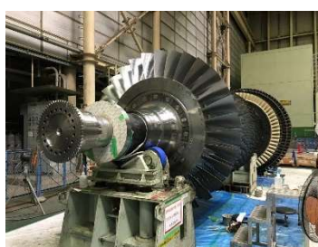
Placing new gas turbine temporary before installation
