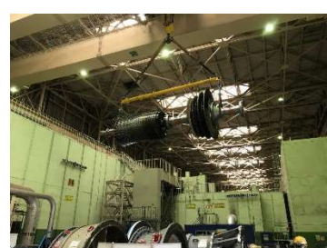
Lifting new gas turbine rotors
