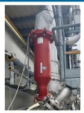
Detects the pressure wave of the primary explosion and immediately sprays fire extinguishing agent to prevent secondary explosions
