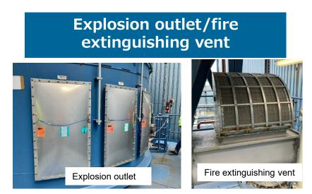
Prevents damage to equipment by releasing the pressure from the primary explosion through the outlet Extinguishing vents prevent flame loss
