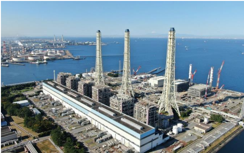
Anegasaki Thermal Power Station, which contributed to electricity supply-demand in a supply capacity through a successful bid in the "Public Auction for Additional FY2021 Winter Power Capacity" (Unit 5 is second from the right)
