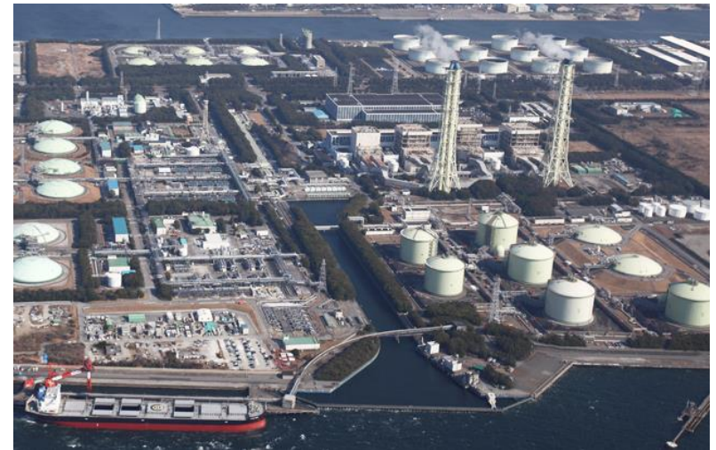
Sodegaura Thermal Power Station (Unit 1 is on the left)
