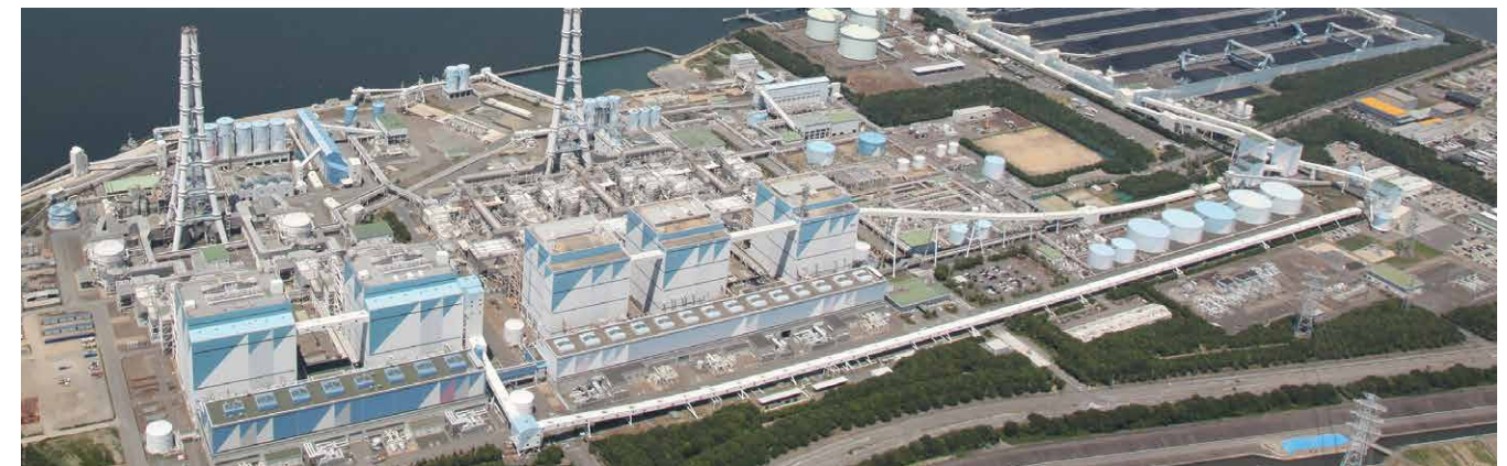
Hekinan Thermal Power Station (Hekinan City, Aichi Prefecture), where the demonstration project related to ammonia co-firing will be conducted
