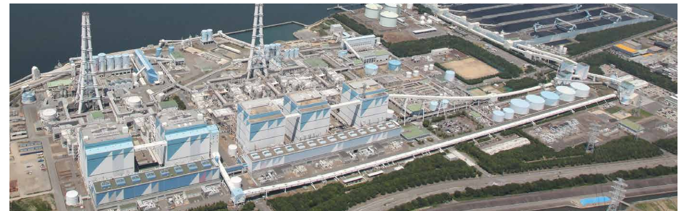
Hekinan Thermal Power Station (Hekinan City, Aichi Prefecture), where the demonstration project related to ammonia co-firing will be conducted
