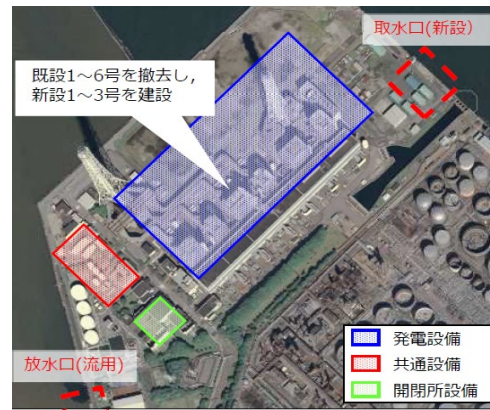
Photo-2 Project 5: JERA Goi Thermal Power Station
