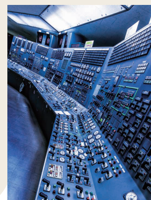
BTG operation panels in the central control room of Units 1 and 2
