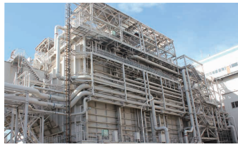
Exhaust gas denitration equipment (removal of NOx)
