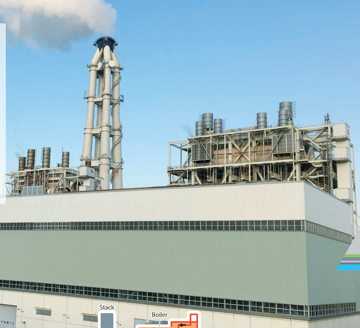
Overall layout of the power station
