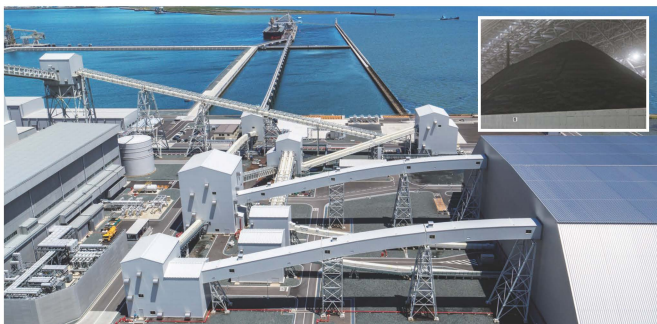
(Center) Enclosed conveyor belts (Right) Indoor coal storage yard
