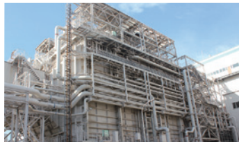
Exhaust gas denitration equipment (removal of NOx)
