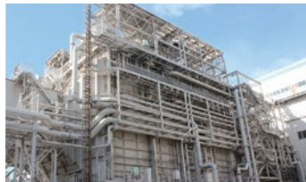
Exhaust gas denitration equipment (removal of NOx)
