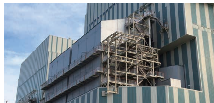
Exhaust gas denitration equipment (removal of NO x )
