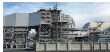
Exhaust gas desulfurization equipment (removal of SO x )
