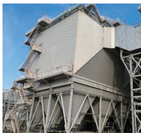
Electrostatic precipitator (removal of soot and dust)
