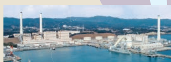
Hirono Thermal Power Station
