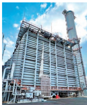
Exhaust gas denitrator (removal of nitrogen oxides (NOx))
