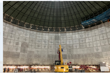
Inside the No. 1 fuel ammonia tank (October 2025)
