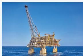
Wheatstone LNG Project, Australia Source: Chevron Australia
