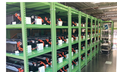
Large-capacity sweep energy storage system that uses electric car batteries
