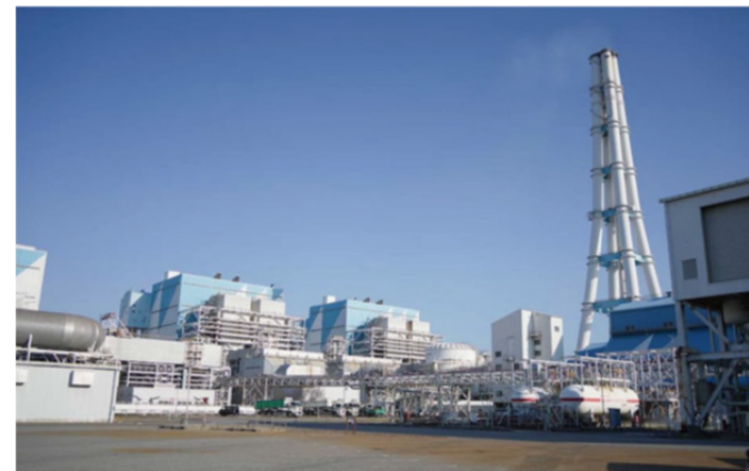
Commercial operation of ammonia fuel substitution at Hekinan Thermal Power Station (Aichi Prefecture)
