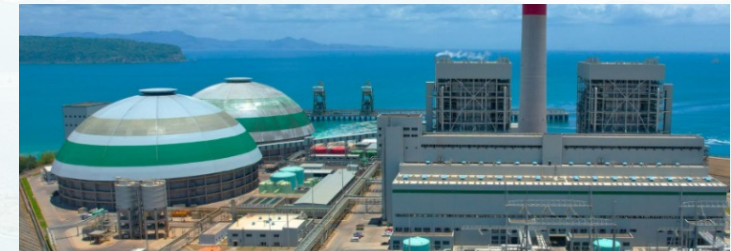
GNPD Power Plant, in which Aboitiz Power holds an equity interest
