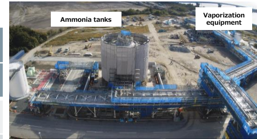
Progress of equipment construction
