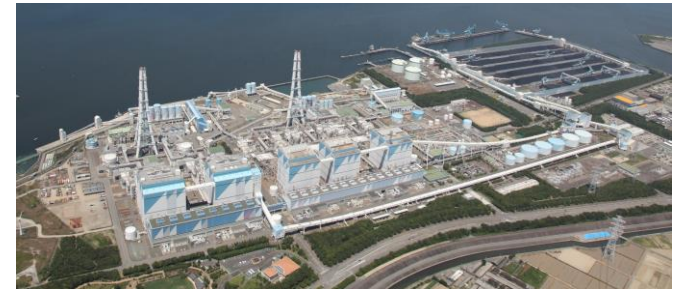
Hekinan Thermal Power Station, a potential candidate site for ammonia co-firing demonstration in actual plants
