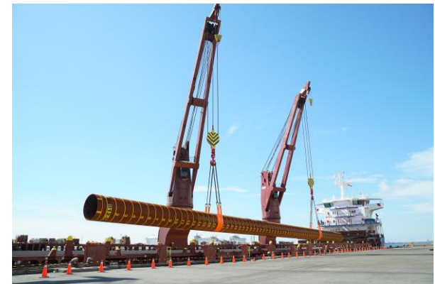
Pin pile for Formosa 2 unloaded in Taichung Port (Provided by Formosa2)
