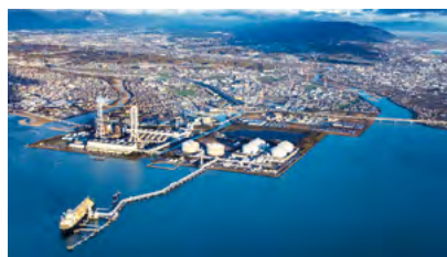
Kawagoe Thermal Power Station
