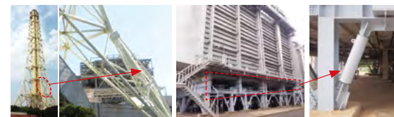
Aseismic reinforcement for chimney at Anegasaki Thermal Power Station
