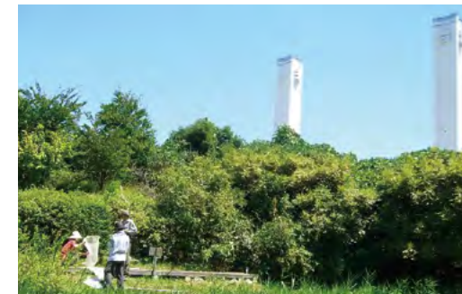
Yokohama Thermal Power Station
