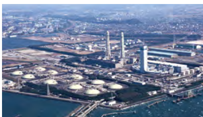
Futtsu Thermal Power Station
