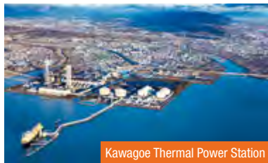
Kawagoe Thermal Power Station
