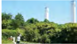
Yokohama Thermal Power Station
