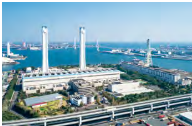
Yokohama Thermal Power Station
