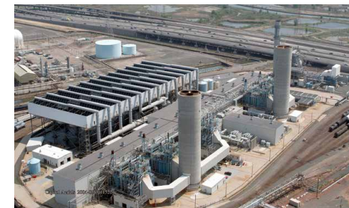
Hydrogen Power-enabled Linden Gas Thermal Power Station Unit 6 (US)
