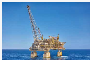
Wheatstone LNG Project, Australia Source: Chevron Australia
